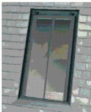
**Rooflights, where used, should be of a suitable conservation type, with a vertical glazing bar and set as low as possible in the plane of the roof as illustrated above**
