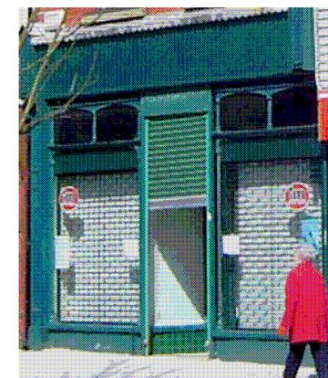
A lattice brick shutter (preferably internal) provides a much more subtle feature than a bulky solid roller shutter.
