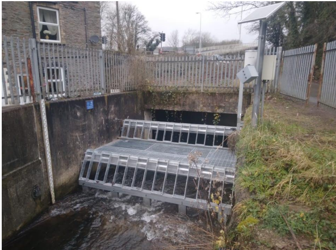
Culvert Inlet Upgrade – Nant Cae Dudwg Flood Alleviation Scheme 2024 January 2024
