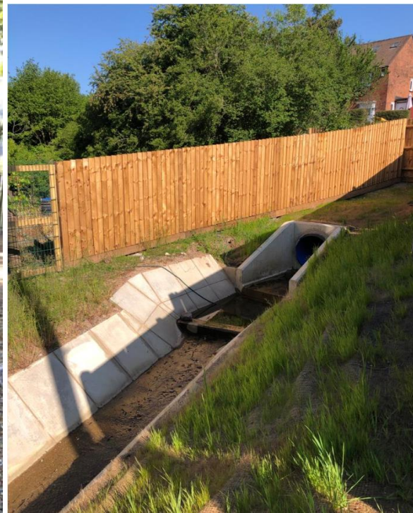
Culvert improvements carried out as part of the Treorchy Flood Alleviation Scheme Phase 1
