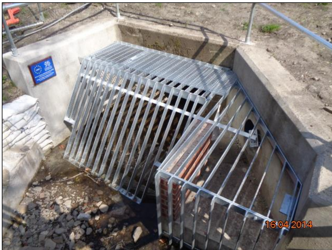
Culvert Inlet Upgrade - Nant Gwar Phase 1 Flood Alleviation Scheme, Aberaman
