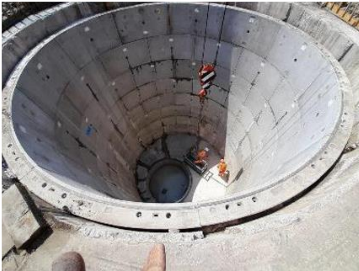
Image of Glenboi Pumping Station under construction.
