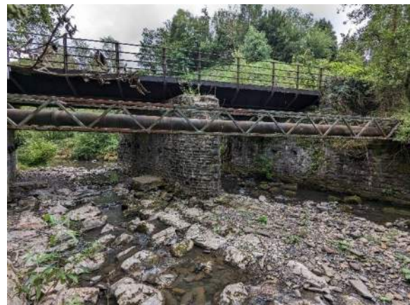
Figure 35 - Tylerstown south bridge.
