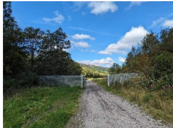
Figure 25 - Gated fence at north of Phase 5.
