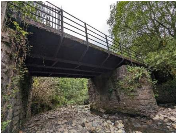
Figure 30 - Tylerstown north bridge.
