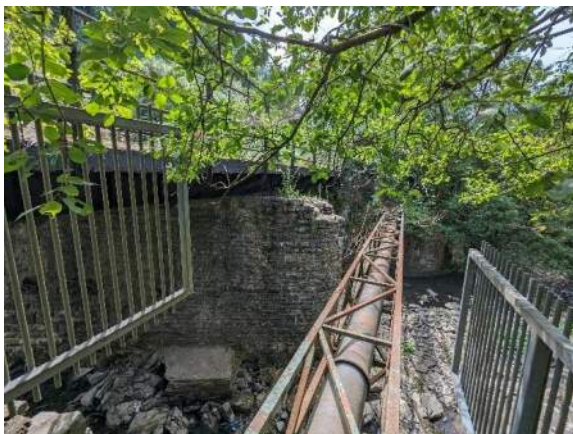
Figure 34 - Tylerstown south bridge.
