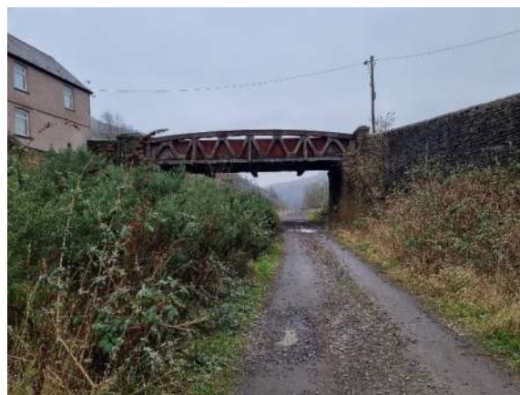
Figure 12 - Bridge at Blaenllechau (not subject to works).
