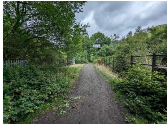
Figure 31 - Tylerstown north bridge
