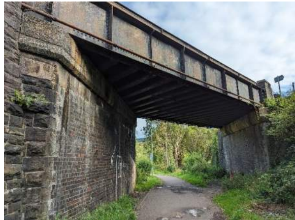
Figure 37 - Road bridge at entrance at south entrance to Phase 5.
