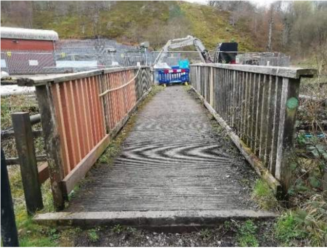
Figure 26 – footbridge over river
