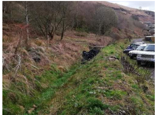
Figure 23 ditch running along eastern side of path. Note parked cars
