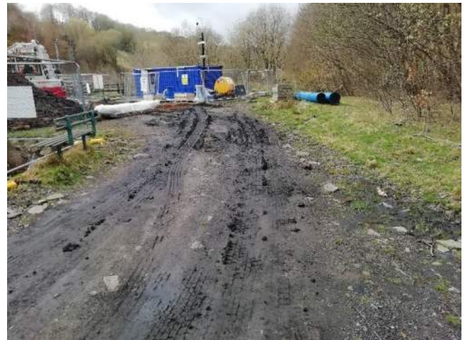
Figure 25 – approach to works site and small footbridge
