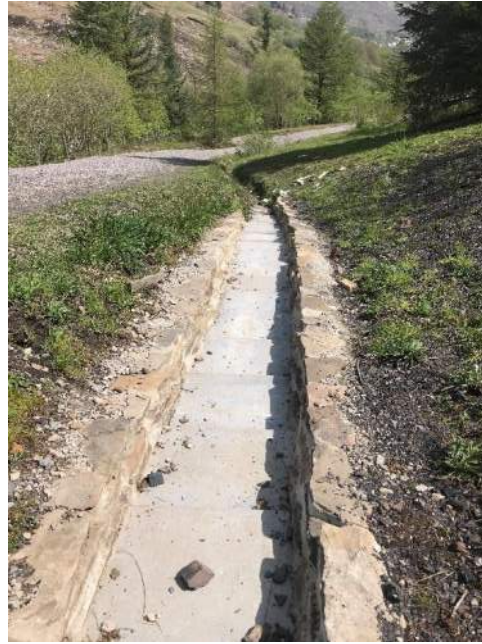
Figure 33 – new concrete drainage
