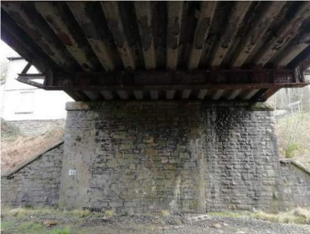
Figure 20 – under road bridge with bat features on wall top
