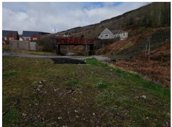
Figure 19 – approaching road bridge
