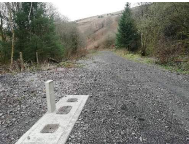
Figure 12 – new concreted structure in path
