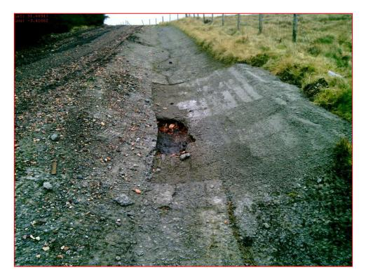
Figure 3.11 Upper sections of Channel 2. Concrete channel with visible damage.
