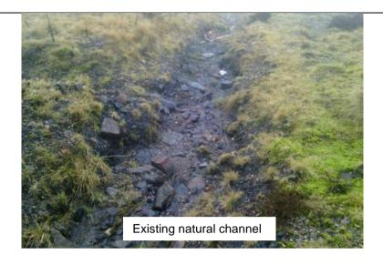
• To the north west of the site there are two natural ditches that collect run-off and discharges to a lower down concrete channel finally discharging to the Afon Rhondda Fach
