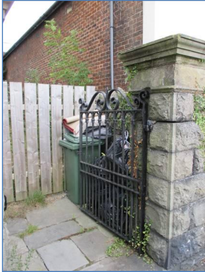
Lack of bin storage can contribute to developments looking untidy
