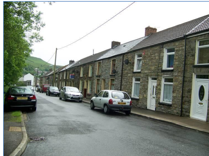
Terraced houses are often not suitable for conversion to flats
