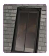
Rooflights, where used, should be of a suitable conservation type, with a vertical glazing bar and set as low as possible in the plane of the roof as illustrated above
