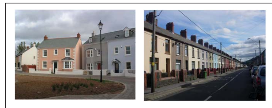
Above right - no dormers would be appropriate on the front of this terrace due to the visual impact of breaking the consistent roofline. Above left - additional appropriately designed dormers may be acceptable here due to the varied rooflines and the existing presence of dormers.
