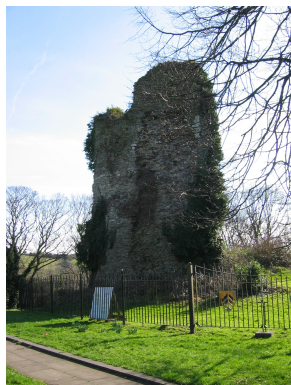
Photo 3.1 The Castle Raven Tower (2005)
