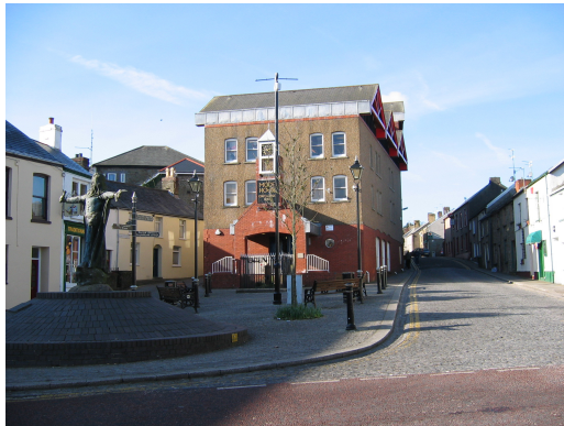
Photo 2-24 The Model House Craft & Design Centre: This was originally built as a workhouse in 1784, and then became a public house, a grocers and later a general store, and a glove manufacturing factory until the late 1960's. It then stood empty for some years before being bought by the local authority and converted in 1989. It has now become an award-winning contemporary craftwork gallery and shop, with fifteen studio workshops for local artists provided on the upper floors. The Centre is open Tuesday-Sundays (10am –5pm) and on bank holidays, and currently hosts contemporary craft exhibitions (including glass, ceramics, jewellery and textiles), with a gift shop and permanent exhibition of Royal Mint coining, and craft workshops for adults and children. A total of 38,000 visitors were recorded in 2004. The rear of the Model House building is occupied by Llantrisant Library, which is contained in a separate unit without access into the main building.
