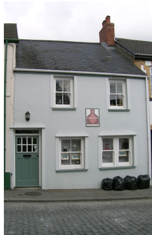
Photo 2-22 The Pottery on Swan Street, Photo 2-23 facing the Bull Ring: Another sensitive renovation of timber fenestration reflective of the building's original style, although it would not have been rendered and the signage is not sympathetic to the building's original character.
