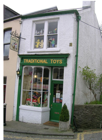
Shop on George Street, facing the Bull Ring: The façade of this building has changed very little since 1910. A recent renovation has sensitively restored the original signage, timber fenestration and original shop front. However, the original building was not rendered.
