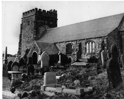
Photo 2-2 Church of St Illtyd, St Gwynno and St Dyfodwg (1967)
