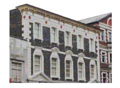
In Pontypridd, there is a greater use of parapet walls, although the roof coverings behind them still need regular monitoring and maintenance.
