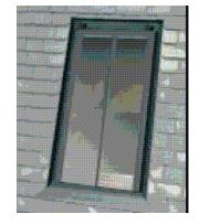
Rooflights, where used, should be of a suitable conservation type, with a vertical glazing bar and set as low as possible in the plane of the roof as illustrated above
