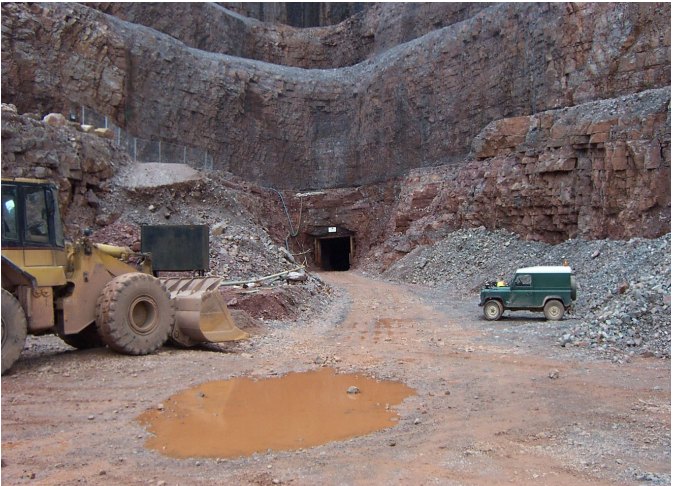
New Tunnel, Taffs Wells Quarry, Cardiff
