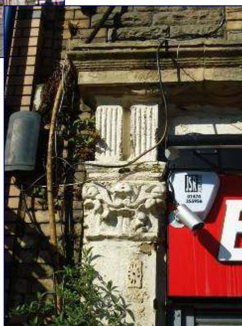
An example where original, ornate shopfront features survive but suffer from poor maintenance, excessive cables and wiring and unsympathetic signage
