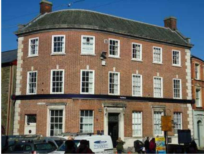
The grade II listed NatWest Bank, where a mixture of brick, stone and natural slate has been used to great effect, with original timber windows surviving.
