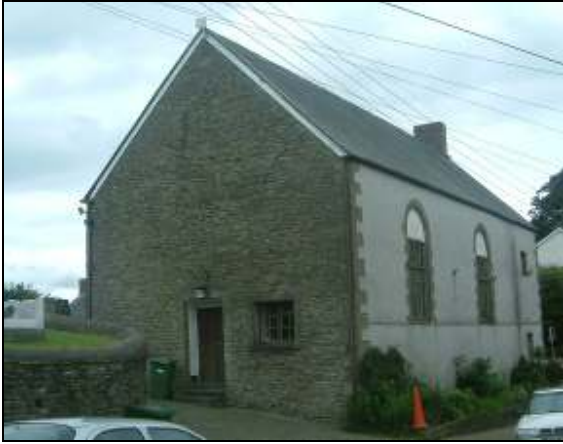
Church Hall, Swan Street
