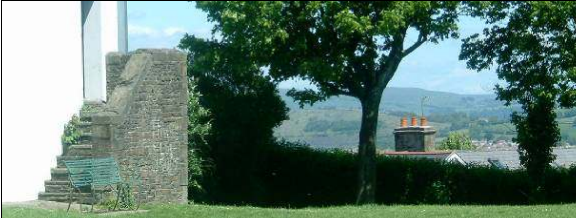
View east across Castle Green showing the dramatic impact of the long distance outlook and importance of managing tree growth to retain these views
