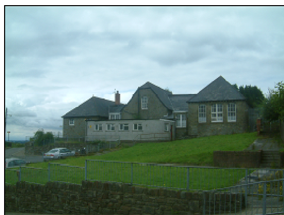
Old primary school, School Street, closed in 2005, an attractive Victorian building, offering opportunities for re-use.
