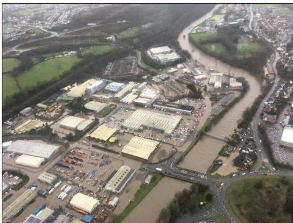
Figure 3: Aerial view of Treforest Industrial Estate and Upper Boat following Storm Dennis (Image: National Police Air Service)
