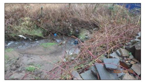
Figure 5: Evidence of submerged 'Culvert Inlet 1' which surcharged during Storm Dennis (captured by RCT's Flood Risk Management team on 18<sup>th</sup> February 2021)
