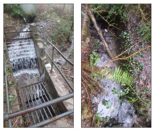
Figure 10: 'Culvert Inlet 5' (left) and 'Culvert Inlet 6' (right) located to the rear of Tyn-y-coedcae which surcharged during Storm Dennis (captured by RCT's Flood Risk Management team on 19<sup>th</sup> February 2020)
