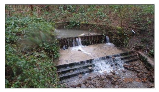
Figure 22: Photo of debris deposition behind the upper debris screen of the Nant Coedcaetylefforest ordinary watercourse (captured by RCT's Flood Risk Management team on 19/02/2020)
