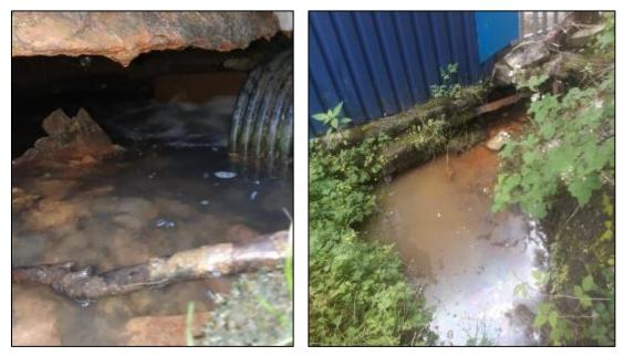
Figure 13: Outfall pipe entering 'Culvert Inlet 2' (left) and standing water surrounding 'Culvert Inlet 2' (right) (captured during CCTV survey operations on 30/06/2020)
