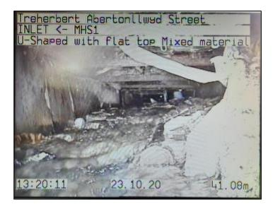
Figure 14: Internal view of 'Abertonllwyd Street Culvert Network 1' looking up towards 'Culvert Inlet 2' (CCTV survey footage captured 23/10/2020)
