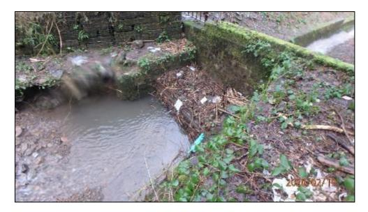
**Figure 23**: Photo of debris accumulation in the upper reaches of the Nant Coedcaetylefforest ordinary watercourse (below the A4061) (captured by RCT's Flood Risk Management team on 19/02/2020)
