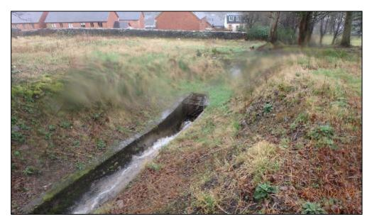
Figure 24: Culvert inlet at Area 2 which conveys the Nant Coedcaetylefforest ordinary watercourse towards Area 3 (captured by RCT's Flood Risk Management team on 19/02/2020)
