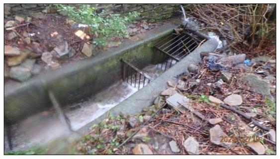
Figure 7: 'Culvert Inlet 3' to the rear of Dumfries Street which surcharged during Storm Dennis (captured by RCT's Flood Risk Management team on 19<sup>th</sup> February 2021)
