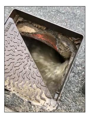
**Figure 10:** Photo of 'Manhole 1' surcharging during Storm Jorje (captured by RCT's Flood Risk Management team on 28<sup>th</sup> February 2020)
