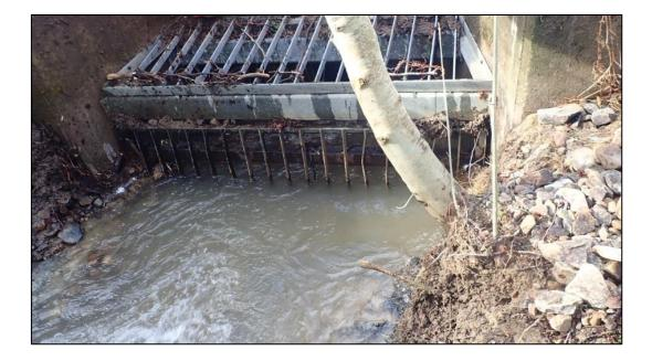
**Figure 18**: Culvert inlet to the rear of Heol Mynydd which surcharged during Storm Dennis due to blockages at the inlet (captured by FRM officers on 17<sup>th</sup> February 2020 following clearance works)
