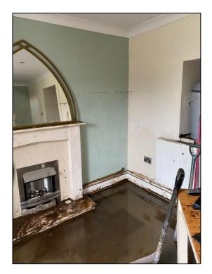
Figure 7: Water depth marks in a property at Cilfynydd Road following Storm Dennis (image provided by resident)
