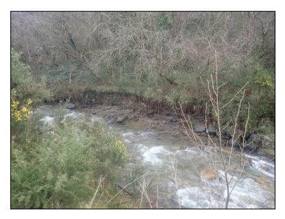
Figure 27: Photo of embankment scour to the Nant Cae Dudwg watercourse (image captured by RCT's Flood Risk Management team on 02/03/2020)
