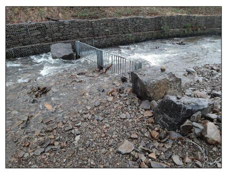
Figure 25: Second upstream debris screen in the Nant Cae Dudwg watercourse captured prior to Storm Dennis
