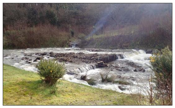
Figure 22: Initial upstream debris screen in the Nant Cae Dudwg watercourse (captured by RCT's Flood Risk Management team on 17<sup>th</sup> February 2020)
