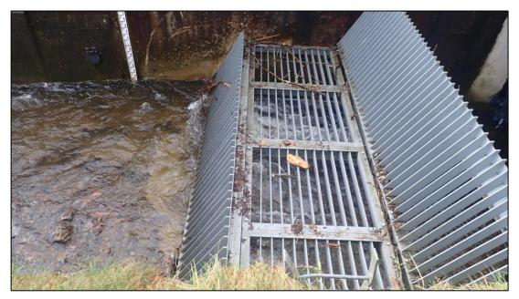
Figure 16: Photo of 'Culvert Inlet 1' (Nant Cae Dudwg culvert inlet) captured by RCT's Flood Risk Management team prior to Storm Dennis on 13<sup>th</sup> February 2020
