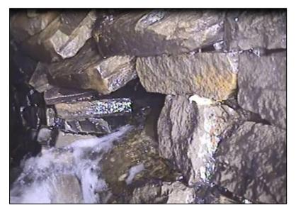
Figure 20: Hole in culvert 22.9 meters downstream of the Ely Brook inlet opposite Royal Oak Inn
