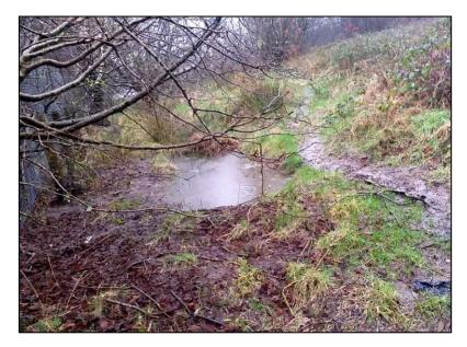
Figure 32: Photo of the drainage ditch overtopping (image captured by resident on 16/02/2020)
