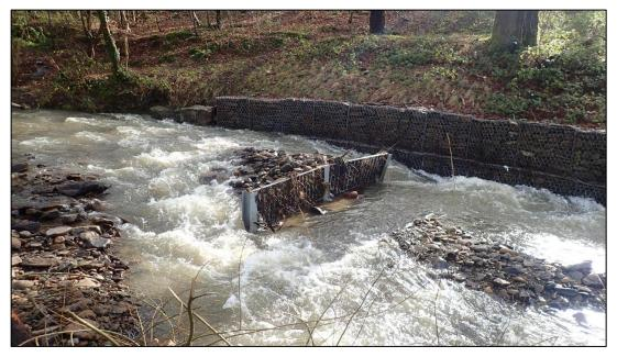
Figure 23: Second upstream debris screen in the Nant Cae Dudwg watercourse (captured by RCT's Flood Risk Management team on 17<sup>th</sup> February 2020)
