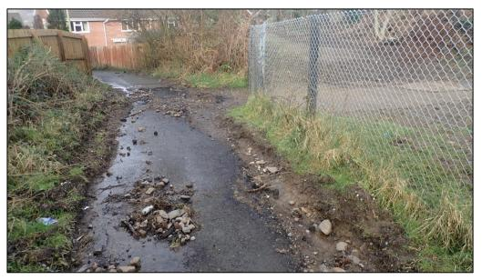
**Figure 12**: Evidence of deposited debris and damages to the bottom of the path looking down towards Brynderwen. Overland flows were observed flowing through land to the right behind the fencing (captured by FRM officers on 17<sup>th</sup> February 2020).
