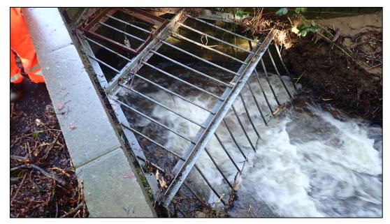
Figure 19: Ely Brook culvert inlet to the rear of Pontshonnorton Road which surcharged during Storm Dennis due to blockages at the inlet (captured by FRM officers on 17<sup>th</sup> February 2020 following clearance works)
