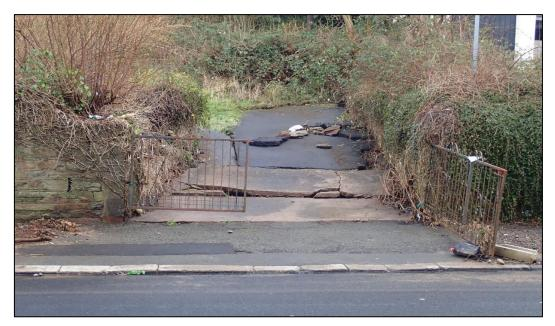
Figure 14: Damages to the driveway situated below the Ely Brook culvert inlet showing evidence of subterranean hydraulic pressure (captured by FRM officers on 17<sup>th</sup> February 2020)
