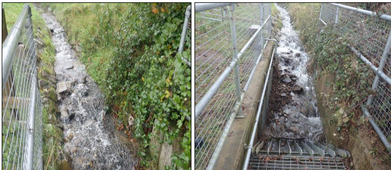
Figure 17: Upstream view of 'Culvert Inlet 2' before Storm Dennis (left) and post Storm Dennis (right) showing silt and stone deposition within the channel (captured by RCT's Flood Risk Management team)
