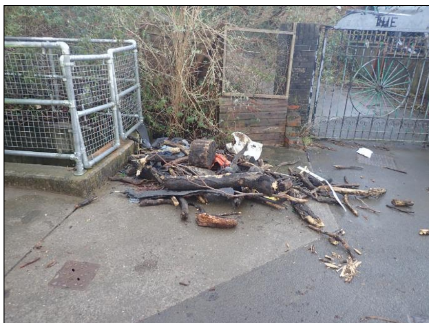
Figure 6: Image of the debris that was cleared from 'Culvert Inlet 1' during emergency cleansing operations (image captured by RCT's Flood Risk Management team on 17 th February 2020)
