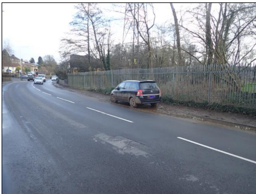
Figure 14: Evidence of mud and silt along the A4054 (Cardiff Road) identified post event as a result of the overtopping of the Nant Lonydd and an ordinary watercourse channel which runs behind the fence (image captured by RCT's Flood Risk Management team on 17 th February 2020)
