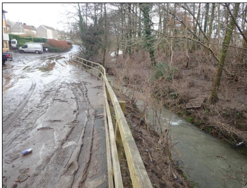
Figure 28: Mud and silt deposited adjacent to Melin Corrwg Business Park as a result of the Nant Lonydd ordinary watercourse overtopping (captured by RCT's Flood Risk Management team on 17 th February 2020)
