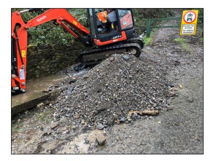
Figure 23: Silt and stone removed from the culvert inlets located upstream of the collapse at 'Culvert Section 2' along Cefnpennar Road (captured by RCT's FRM team on 18/02/2020)
