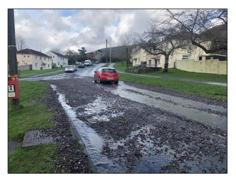
Figure 34: Debris deposited along Bro Deg by the surcharging ordinary watercourse and surface water flows during the storm event (image provided by resident)
