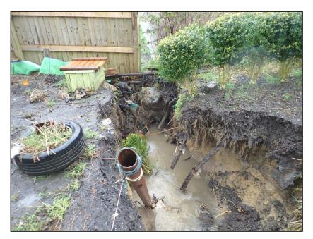
Figure 5: Collapsed culvert in the rear garden of Maeshyfryd identified by RCT's Flood Risk Management team on 10/02/2020
