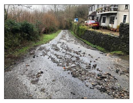
Figure 35: Debris deposited along Cefnpennar Road by surcharging watercourse and surface water flows during the storm event (image provided by resident)
