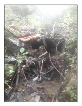
**Figure 28**: Woody debris and other material within the section of ordinary watercourse upstream of 'Culvert Inlet 1' at Tirfounder Road (captured during post event CCTV survey operations)
