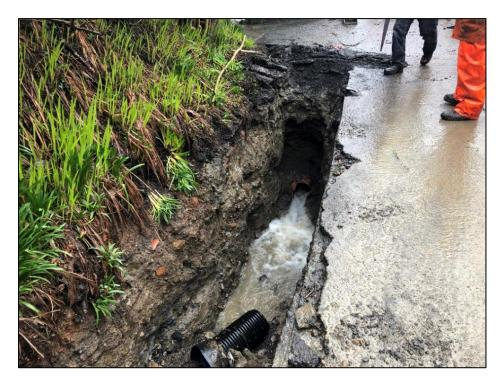
Figure 11: Collapsed culvert network ('Culvert Section 2') to the north of Cefnpennar Road identified during post event inspections (image captured by RCT's Flood Risk Management team on 18<sup>th</sup> February 2020)
