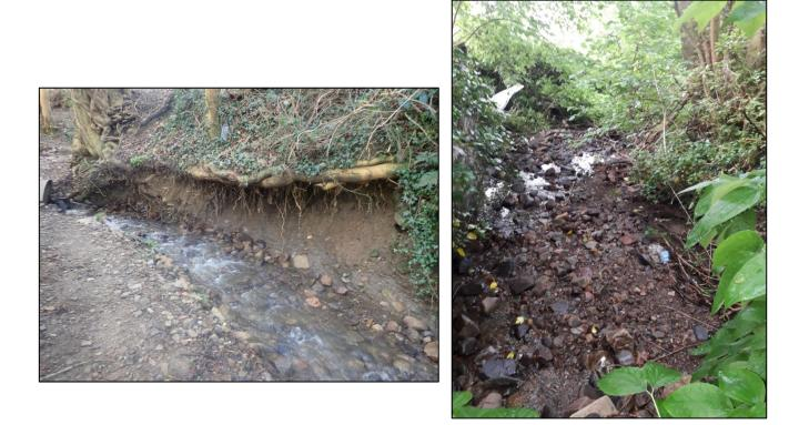
Figure 29: Condition of 'Unnamed Ordinary Watercourse 3' showing significant embankment scour (left) and debris deposition within the channel (right) during post event inspections
