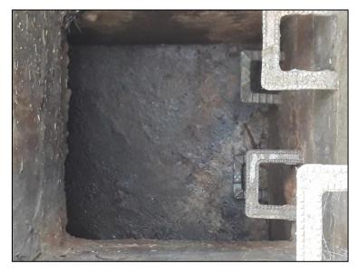
Figure 25: Significant volume of silt identified within 'Manhole 3' during CCTV survey operations (captured in June 2020)
