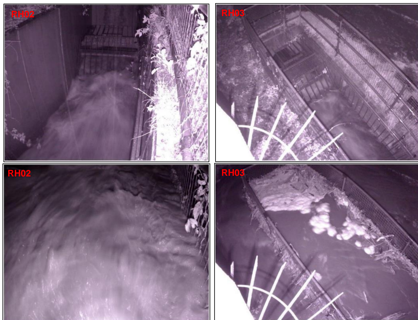
Figure 4: Images captured at RCT's monitoring station at culvert inlets RH02 (left) and RH03 (right) in Rhydyfelin. (04/10/21 22:14 (top left), 04/10/21 23:25 (bottom left), 04/10/21 21:53 (top right), 04/10/21 23:55 (bottom right))
