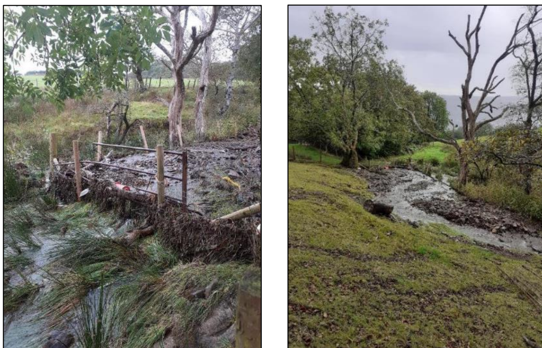
Figure 31: Obstruction of flow (left) and accumulated debris (right) within RH03 Area 3 of 'Unnamed Ordinary Watercourse RH03' (images captured by RCT during post event inspections)
