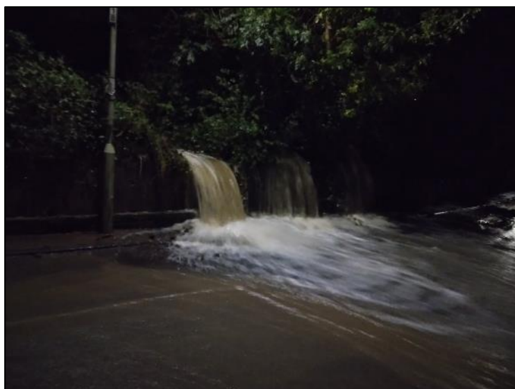
Figure 11: Surcharging flows from 'Culvert Inlet RH02' conveying over the embankment and onto Masefield Way during the storm event (image provided by resident)
