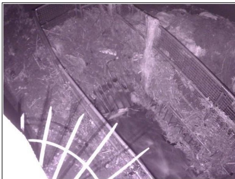
Figure 22: CCTV image of 'Culvert Inlet RH03' captured at 01:57 5 th October 2021
