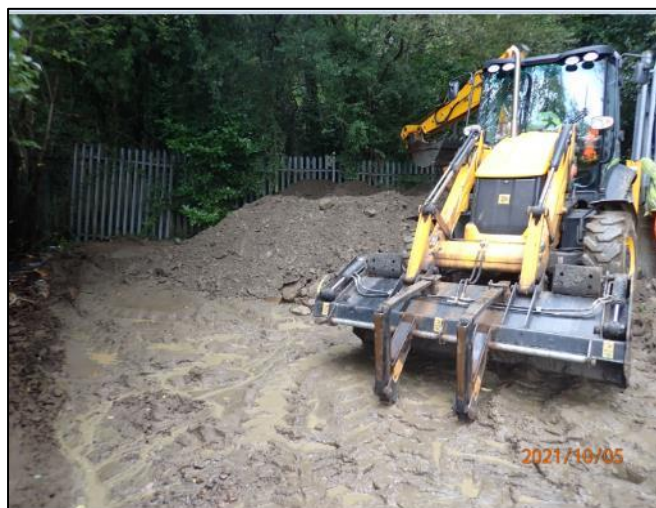
Figure 16: Mud, silt and scour material being cleared from the 'Nant Corrwg Culvert Inlet' by RCT's Highway and Streetcare Depot on 5 th October 2021 (captured by RCT's Flood Risk Management team on 5 th October 2021)
