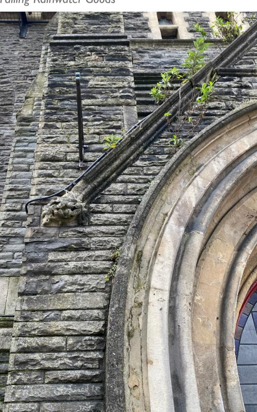
Vegetation Growth to Parapets & Mortar Joints
