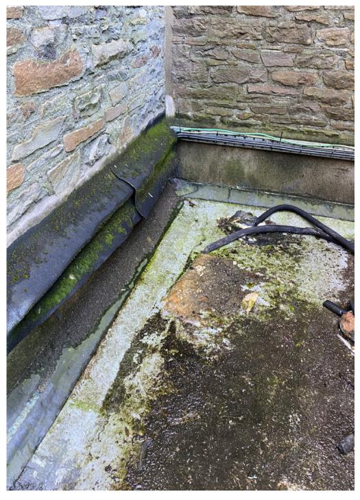
Poor Flashing & Leadwork Details
