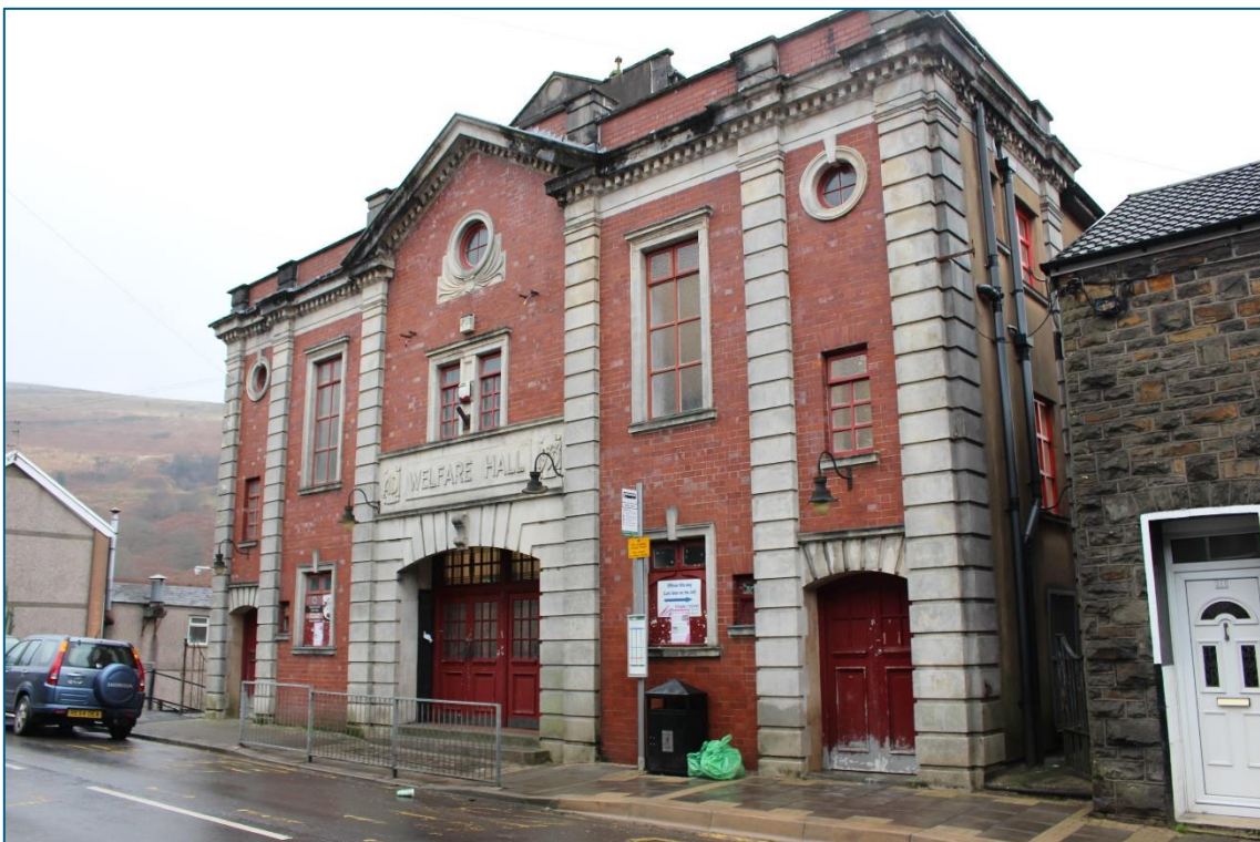
Plate 58. NE facing view of Welfare Hall, Tylorstown (LB18284, NPRN414737)
