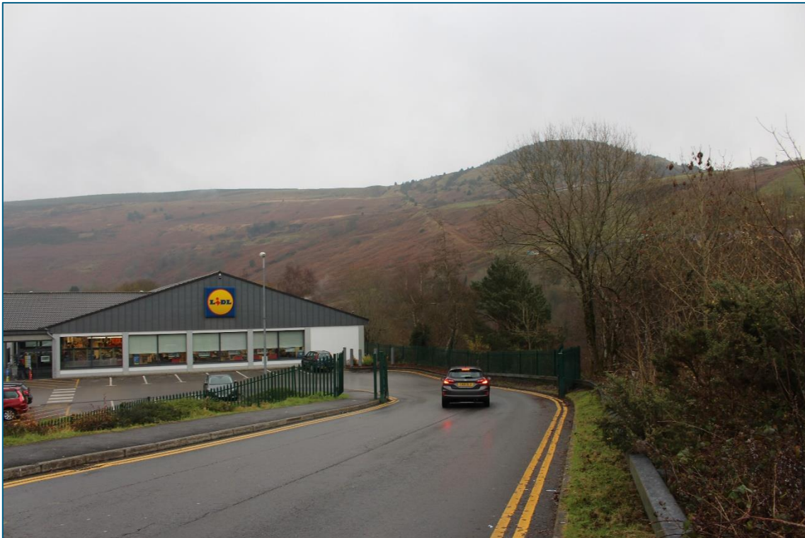
Plate 95. NE facing view of Tramway (TT06) and the Tylors Newydd Tip site (GGAT07879m) from Tylorstown.
