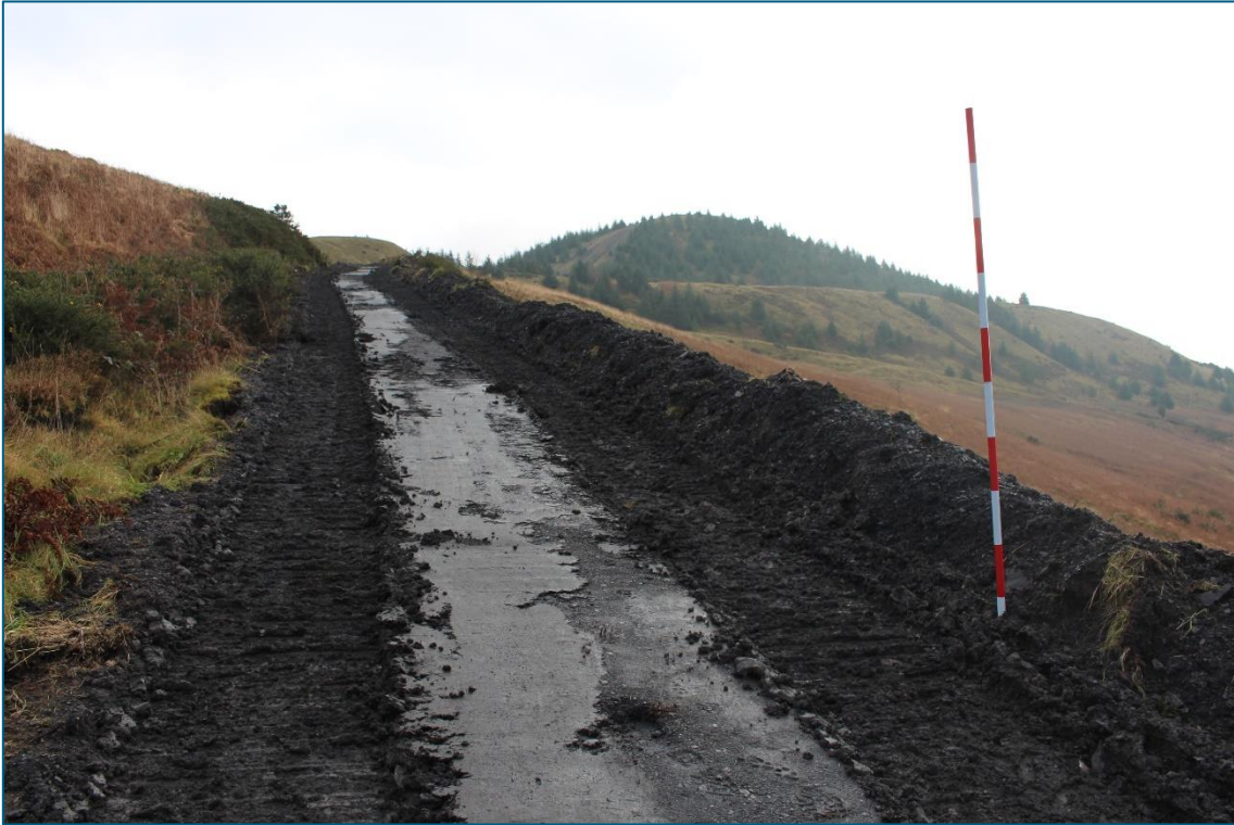
Plate 80. E facing view of Tramway (TT03) showing RH02 'Old Smokey' Tip (TT05) from further down the track.
