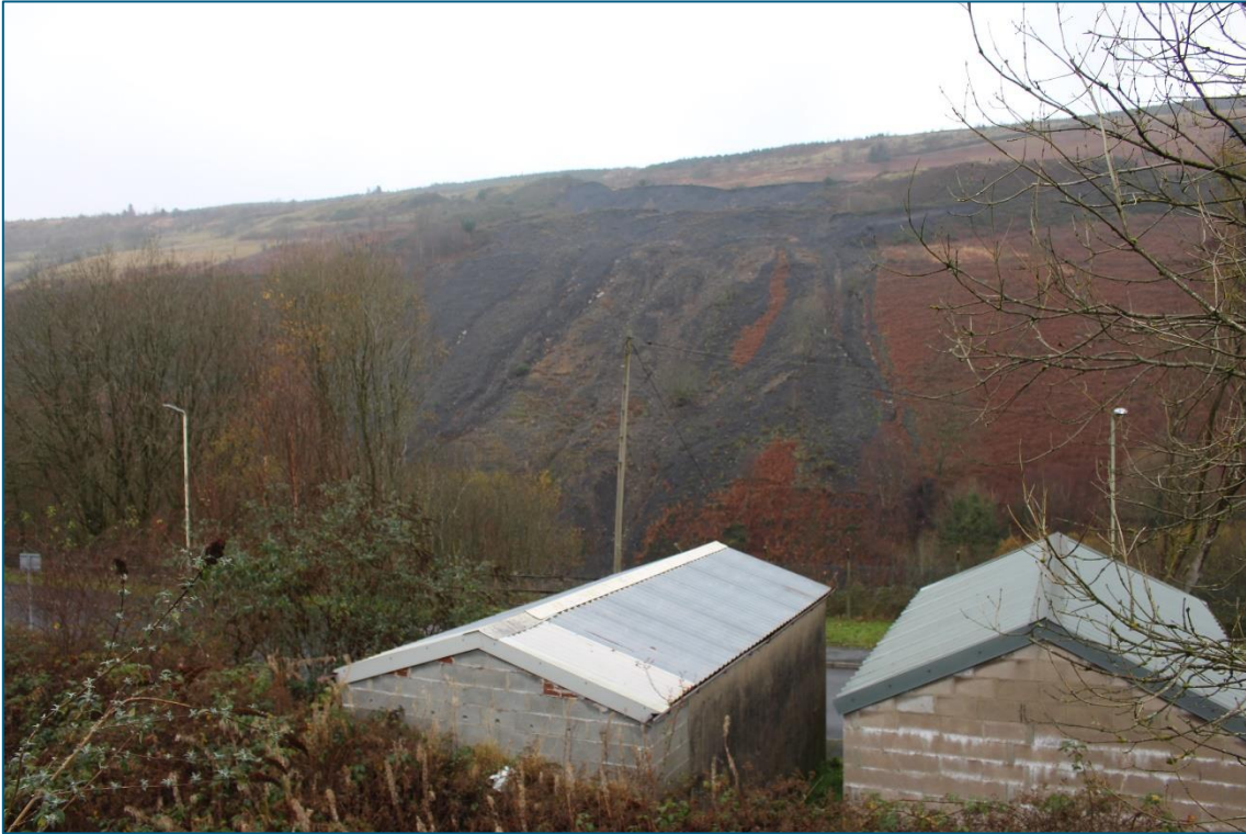
Plate 117. E facing view from HLCA019 'Pontygwaith, Tylorstown & Stanleytown towards RH01 Tylorstown Upper & Lower Tips (TT01 & TT02) showing landslide damage.
