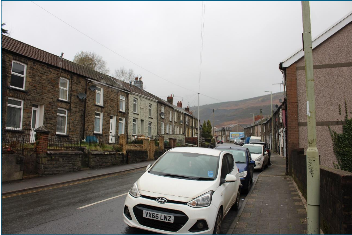
Plate 59. N facing view from frontage of Welfare Hall (LB18284, NPRN414737) towards RH01 Tylorstown Upper & Lower Tips (TT01 & TT02). Here you can see the impact that the landslide damage has had on the setting of the town.
