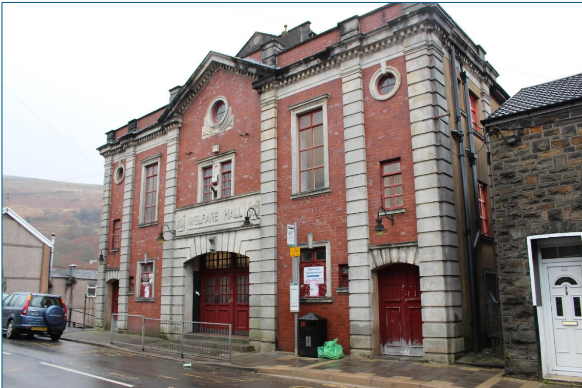
Plate 123. NE facing view of Welfare Hall, Tylorstown (LB18284, NPRN414737)
