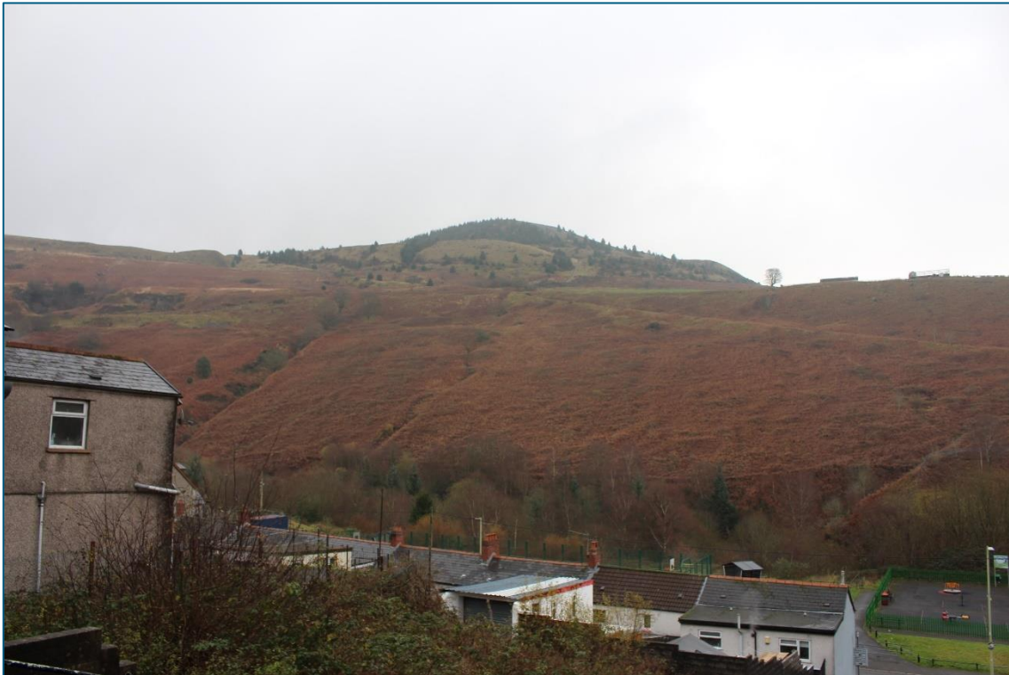
Plate 125. E facing view from adjacent to frontage of Welfare Hall (LB18284, NPRN414737) towards the development site which forms the backdrop of the Listed Building. The Receptor Site is located over the horizon.
