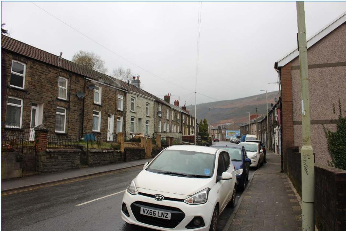
Plate 124. N facing view from frontage of Welfare Hall (LB18284, NPRN414737) towards RH01 Tylorstown Upper & Lower Tips (TT01 & TT02). Here you can see the impact that the landslide damage has had on the setting of the town.
