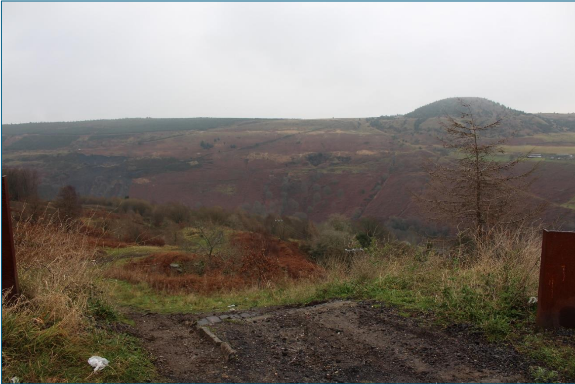
Plate 56. NE facing view from HLCA024 towards RH01 Tylorstown Upper & Lower Tips (TT01 & TT02), Tramway (TT03) and RH02 'Old Smokey' Tip (TT05).
