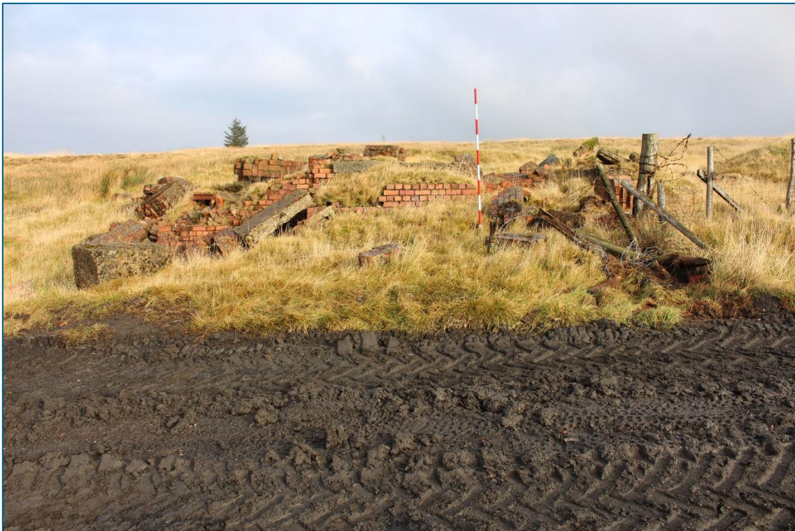
Plate 101. NE facing view of Tramway Winding Engine House (TT07) from intersection of Tramway (TT03) and Tramway (TT06).
