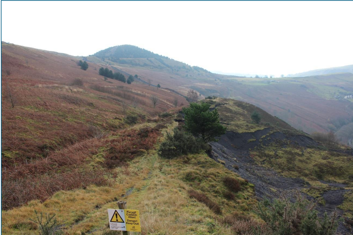
Plate 78. SE facing view of RH01 Tylorstown Upper Tip (TT01) looking towards the development area and showing damage caused by landslide. Tramway (TT03) can be seen in the centre distance.
