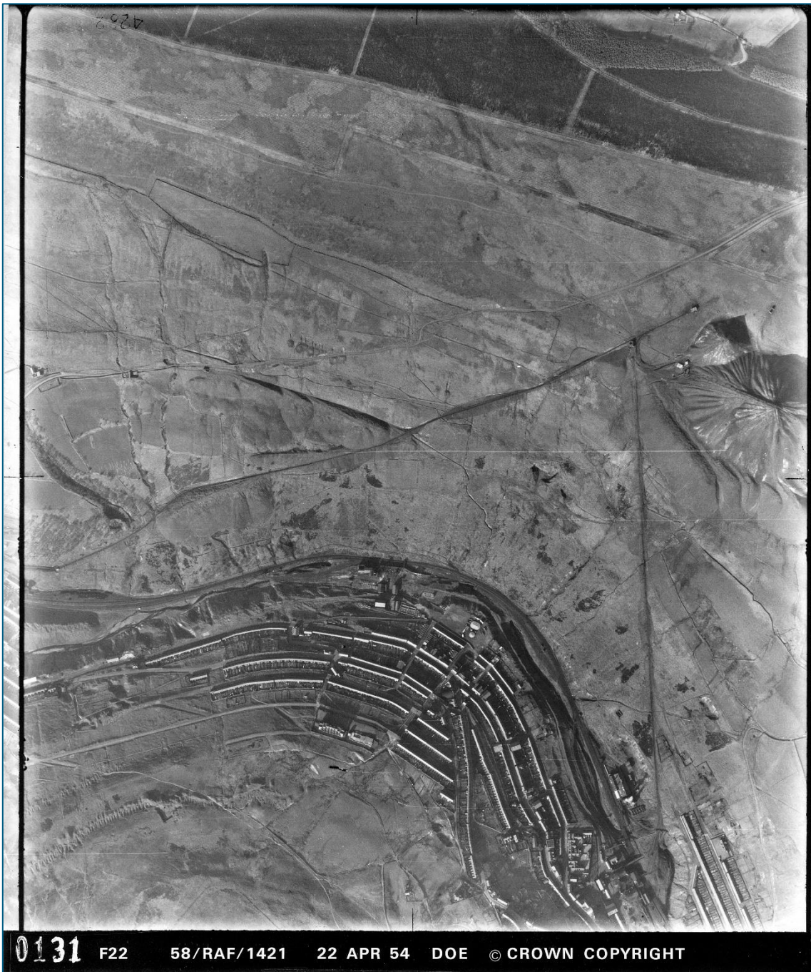
Plate 7. This 1954 aerial photograph really highlights the huge extent of tip material along the valley bottom. ©CRAPW
