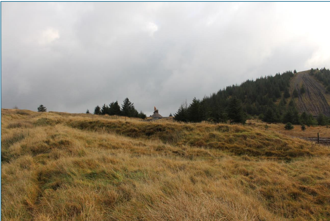
Plate 86. General S facing view of relict section of Tramway (TT03) highlighting surviving earthworks.
