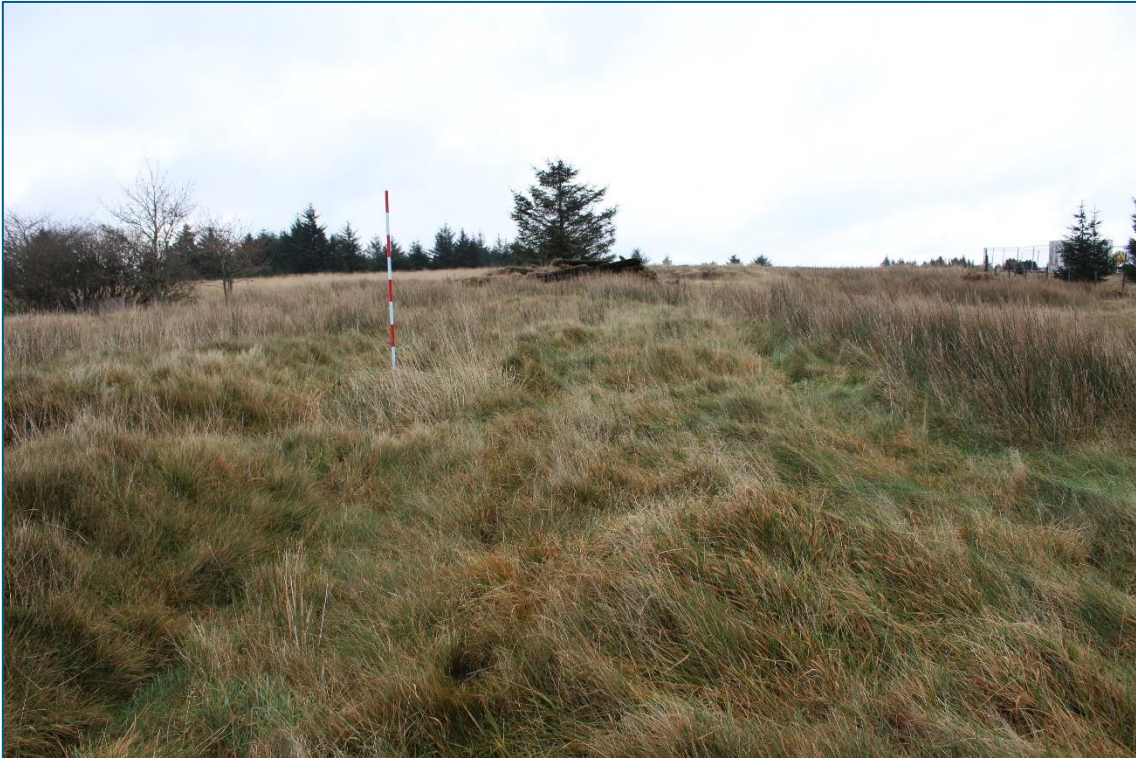
Plate 87. E facing view of relict section of Tramway (TT03) towards Tramway Winding Engine House (TT04) in centre distance.
