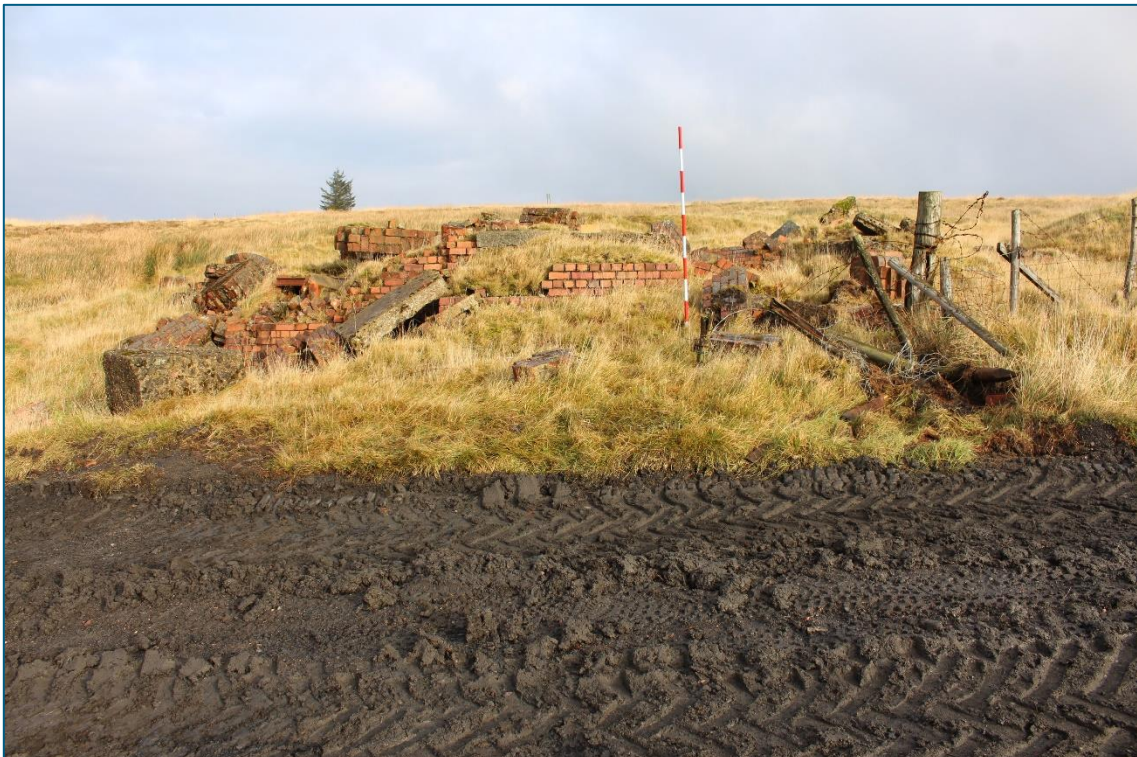
Plate 36. NE facing view of Tramway Winding Engine House (TT07) from intersection of Tramway (TT03) and Tramway (TT06).
