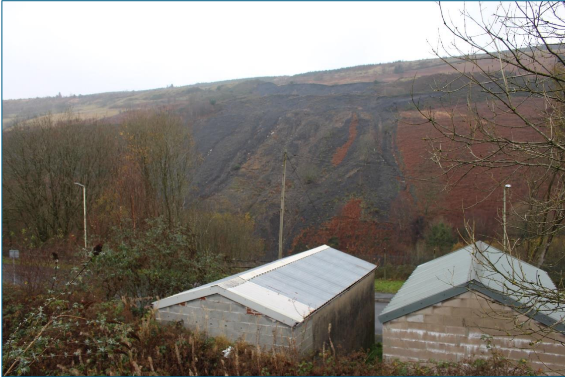
Plate 52. E facing view from HLCA019 'Pontygwaith, Tylorstown & Stanleytown towards RH01 Tylorstown Upper & Lower Tips (TT01 & TT02) showing landslide damage.
