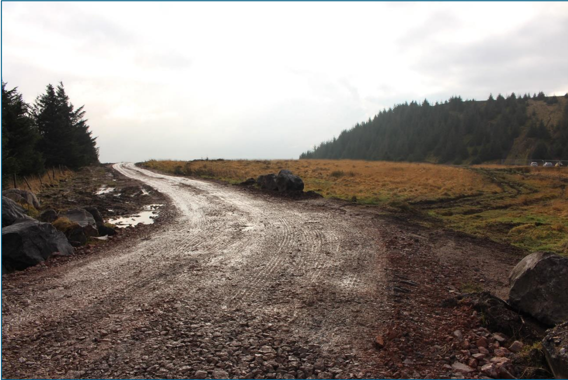
Plate 47. S facing view from current site entrance towards proposed Receptor Site location with RH02 'Old Smokey' Tip (TT05) in the centre right.
