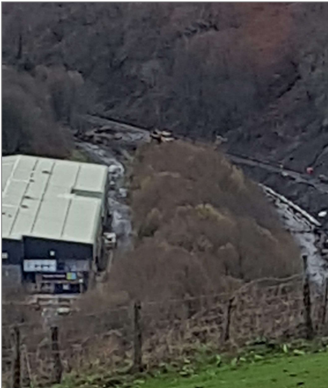
Figure 2: Some Phase 1 activity as seen from Position 2
